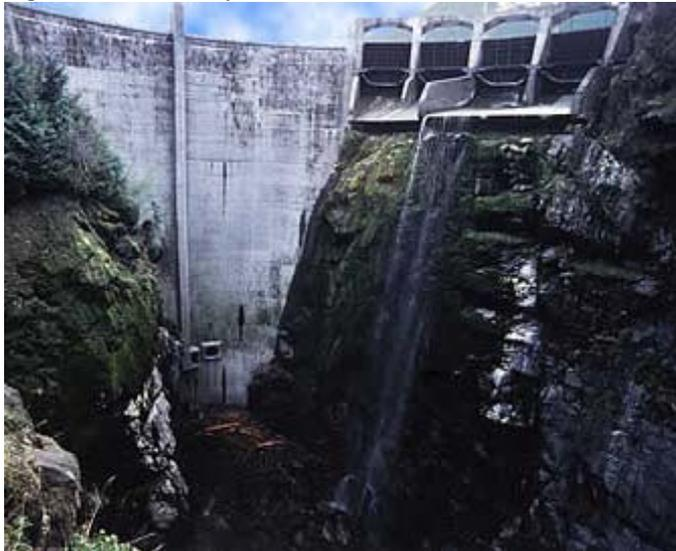
The 33m high Elwha and 65m high Glines Canyon storage dams produce a combined total of 28 MW of electricity, but they also isolate spawning areas in the headwaters of the Elwha River for several threatened fish species. These privately-owned dams were built in 1910 and 1926, predating formation of the Olympic National Park in which they are now located.
