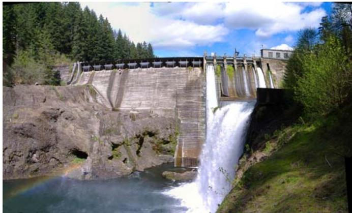
The Condit Dam is a 38m high mass concrete gravity dam and 14.7MW hydroelectric power plant built on the White Salmon River in Washington State in 1913 (Figure 4.4). The dam does not have a fish ladder and blocks fishery access to 22 km of chinook salmon spawning habitat and 53 km of steelhead trout habitat. In addition the reservoir covers 8 km of rapids on a river that is popular with whitewater enthusiasts and
